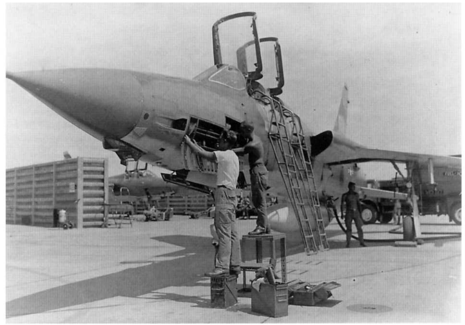
Two ground crewman service the 20MM M61A1 Vulcan cannon on this 388th TFW F-105F at Korat on 17 December 1968. Thunderchief pilots used this weapon for both aerial combat and strafing ground targets. Another crewman supervises the Thunderchief's refueling, standing near the single-point receptacle located on the lower port fuselage. (Cradle of Aviation Museum)
