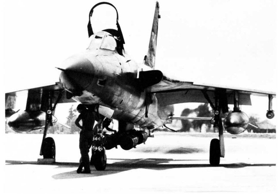
Thuds with diverse ordnance loads. 498 carries 3,000 lb. bombs, used against "hard" targets, while 344 carries cluster bomb units and Mk 81's for use against personnel. Both assigned to 355th TFW at Takhli in 1970. (D.M. Weaver via Jim Farmer)
